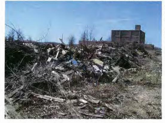
Date: 2 April 2008 Time: 12:20 pm - 1:25 pm Direction: SW Photo by: C. Cahnovsky Exposure #: 037 Comments: Broken concrete, landscape waste, scrap metal, and damaged dimensional lumber near northeast corner of site.
